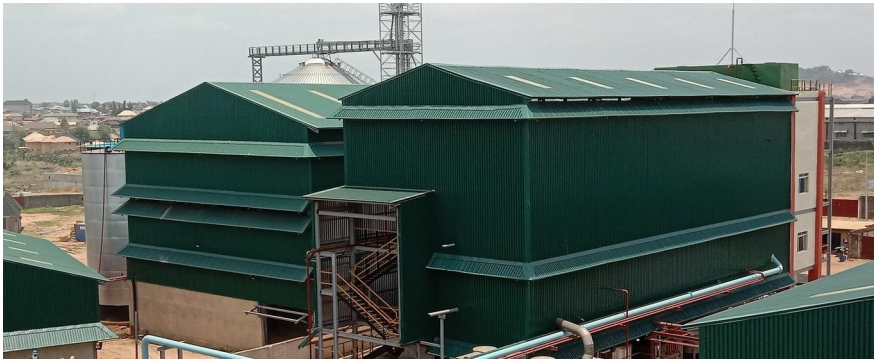
FAME biodiesel plant. Photo: Namindo Pty Ltd.
