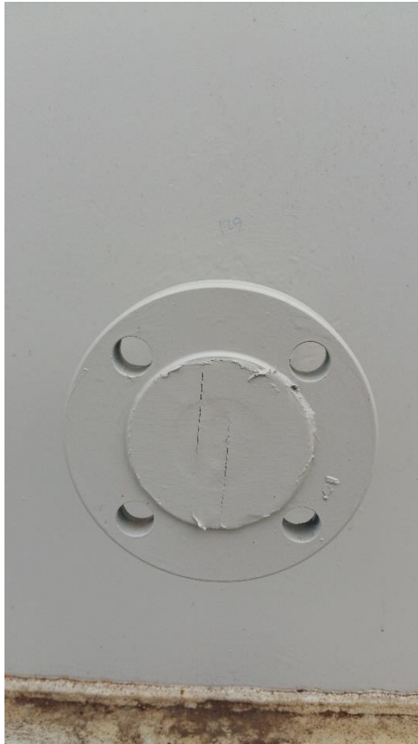
Spare Flange [for Fiber Optic Entrance and Exit] 2" RF 150#
