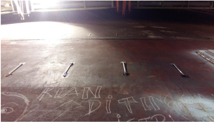
Insulation Anchor [Max Load Per Anchor : 20kg]
